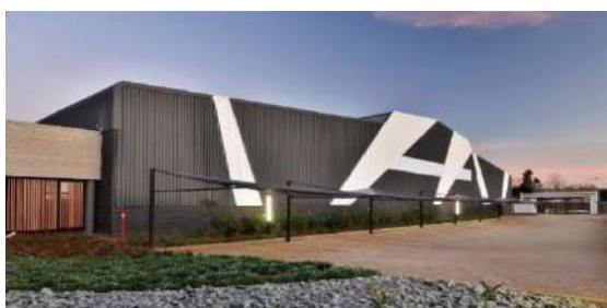
Denver Warehouse (GLA 9 752 m 2 ) Industrial Denver, Johannesburg, Gauteng
